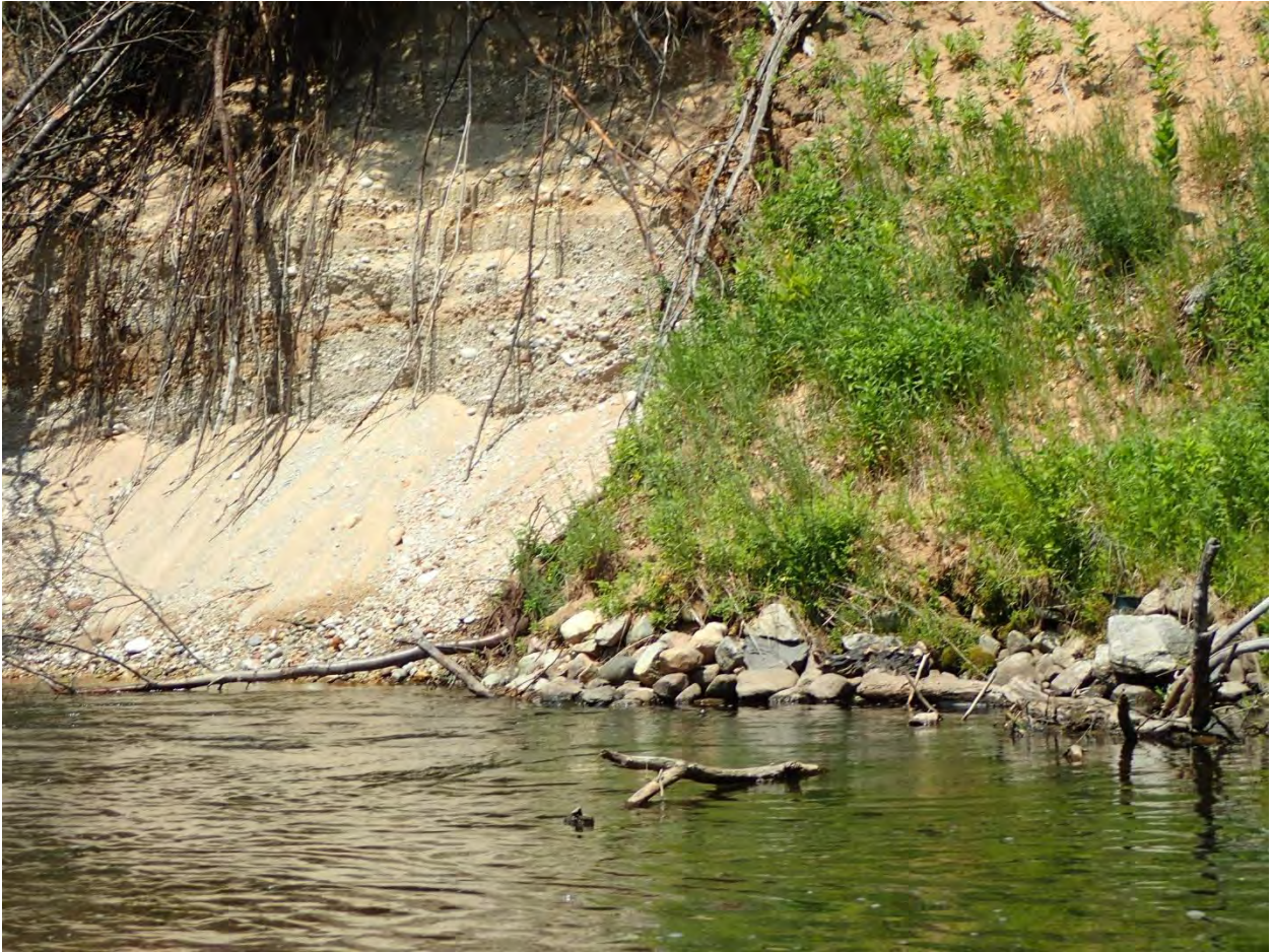
LM#73-2021 (closeup of prior fieldstone stabilization effort)
