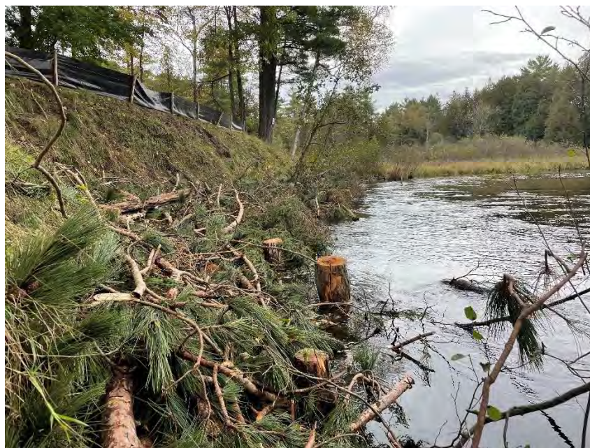
Constructed log jam, Little Manistee River
